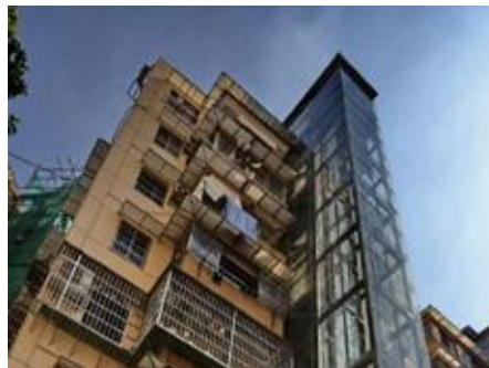
Modernization and Upgrading
